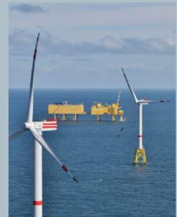
By 2023 TenneT will have realized 17.1 GW of offshore connection capacity (13.3 GW for offshorewind energy, 3.8 GW for interconnection): 13,000 km cable.
